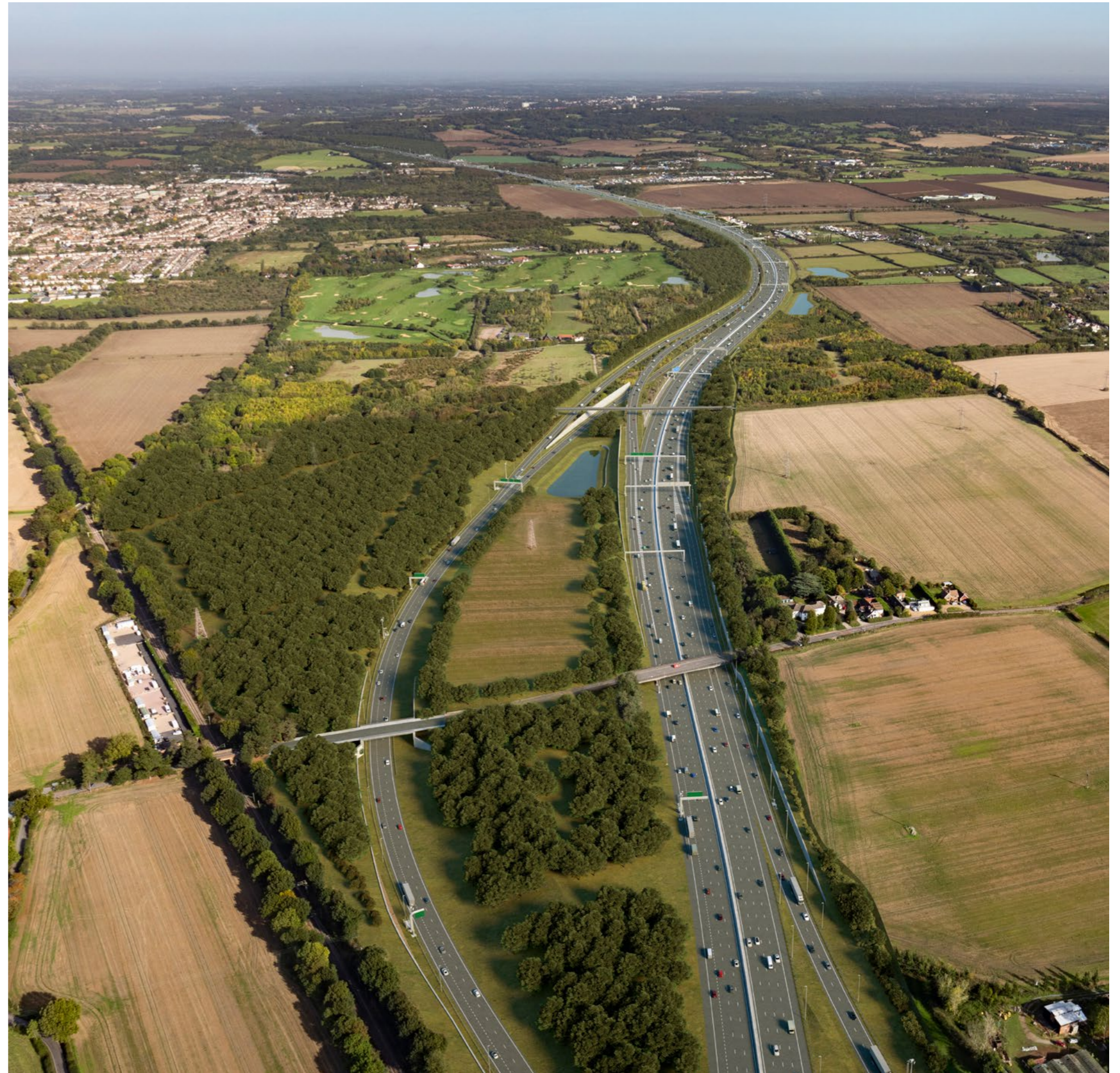
Illustrative view of increased planting and woodland where the Project route meets the M25
