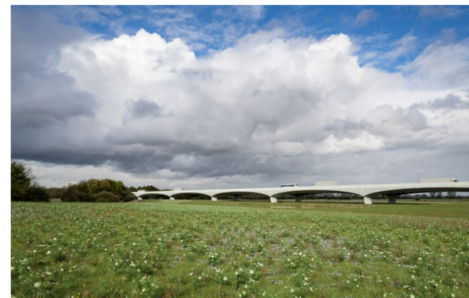
Illustrative view of the Mardyke and Orsett Fen viaducts as they pass through the fenland landscape
